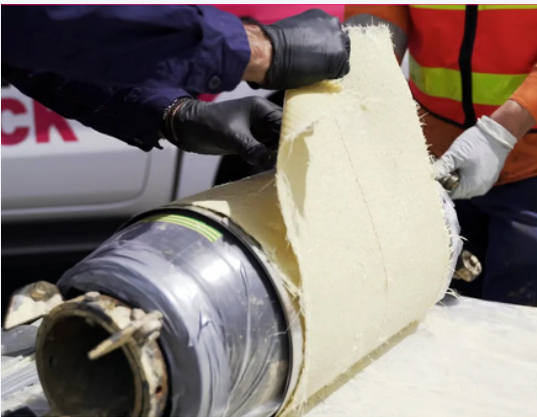
Preparing the seal
