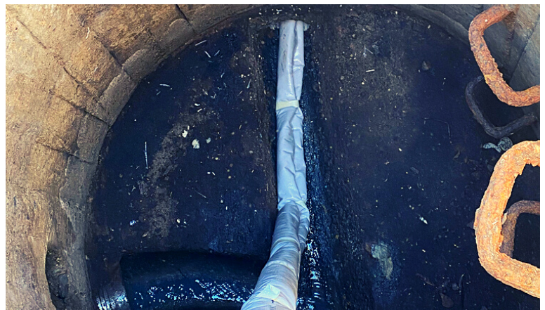
IMPREGNATED LINER INSERTION INTO RETIC
