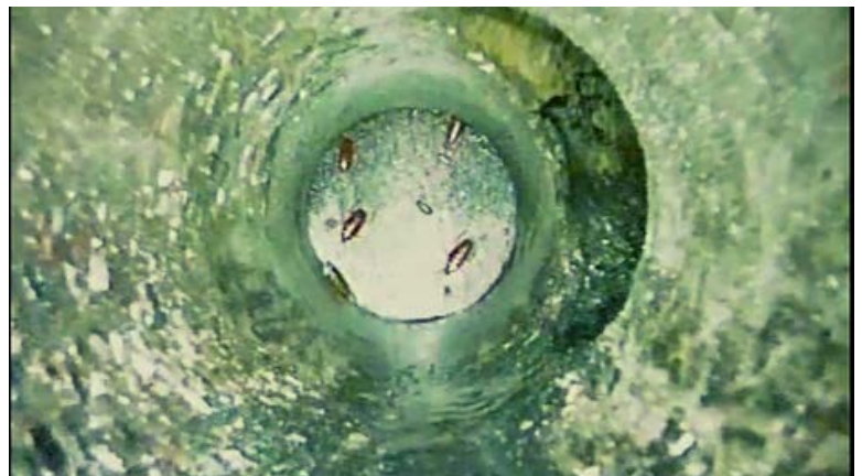
PRE CCTV - LAST JUNCTION BEFORE END OF LINE (EOL)
