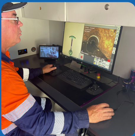
Expert CCTV technology
