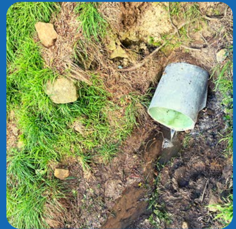
Post Curing at the Outfall
